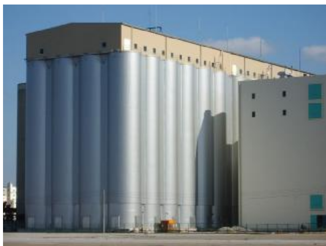
▲ The Completed Chiba Mill Grain Silos
