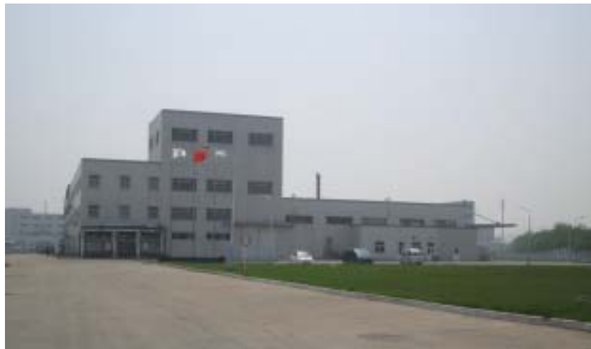
▲ Tianjin Chuan Shun Foods Co., Ltd. (not all buildings shown)
